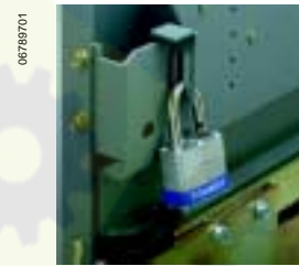
Padlocked Drawout Carriage Hasp
